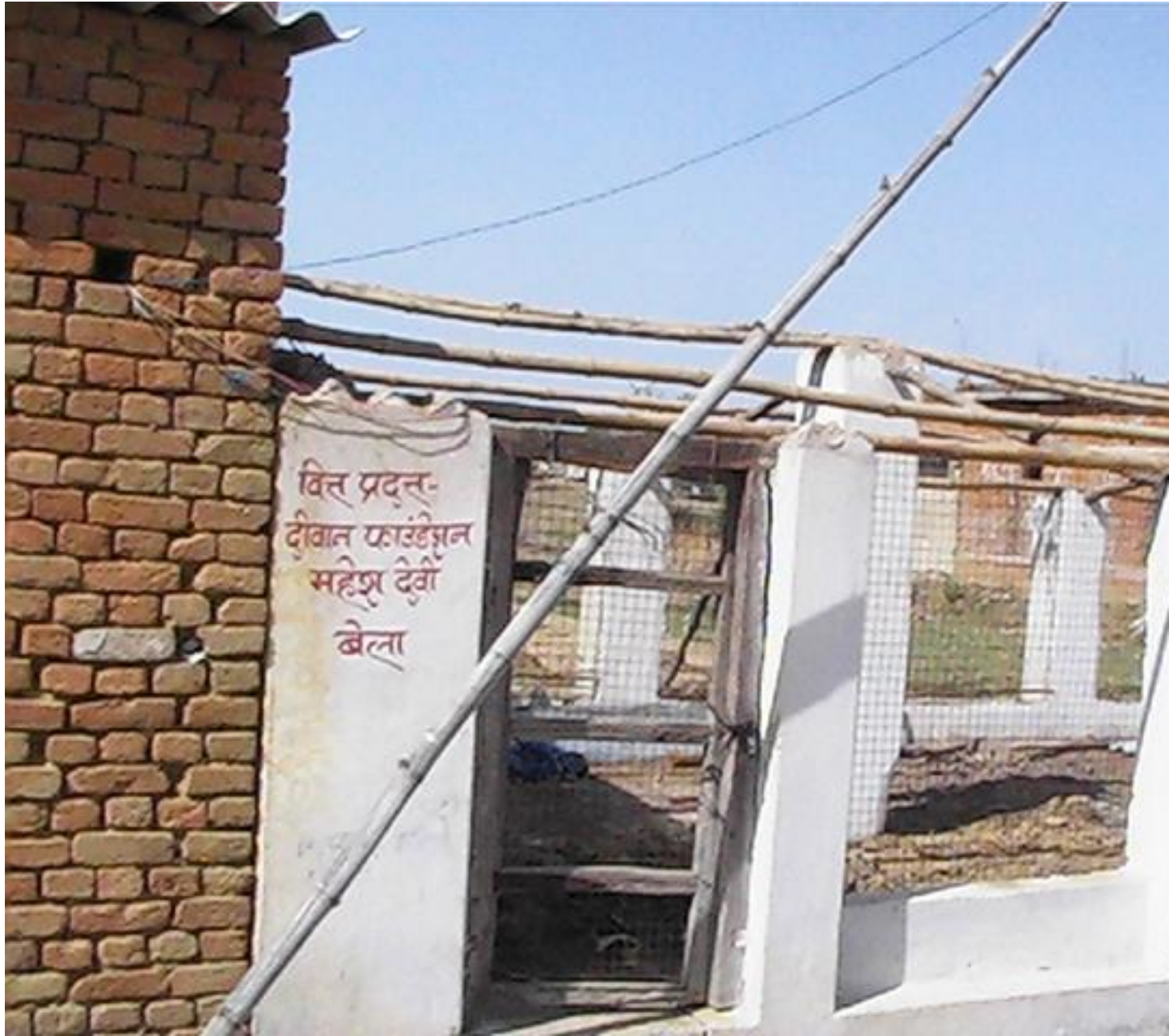
A shed under construction at Bela
